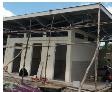
Figure.6 Painting the Wall
