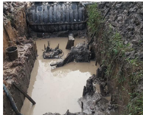
Fig. 2 Fabrication WWTP Installation Work
