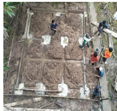
Fig. 4 Foundation Tread Casting
