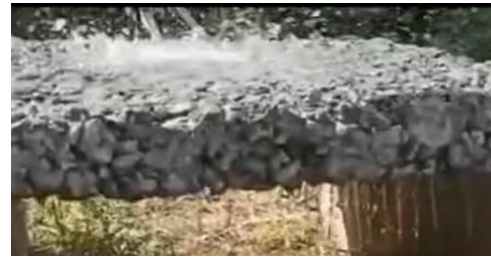
Figure 1. a pervious concrete
