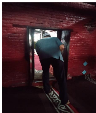
Figure 3. Door on the North Side
